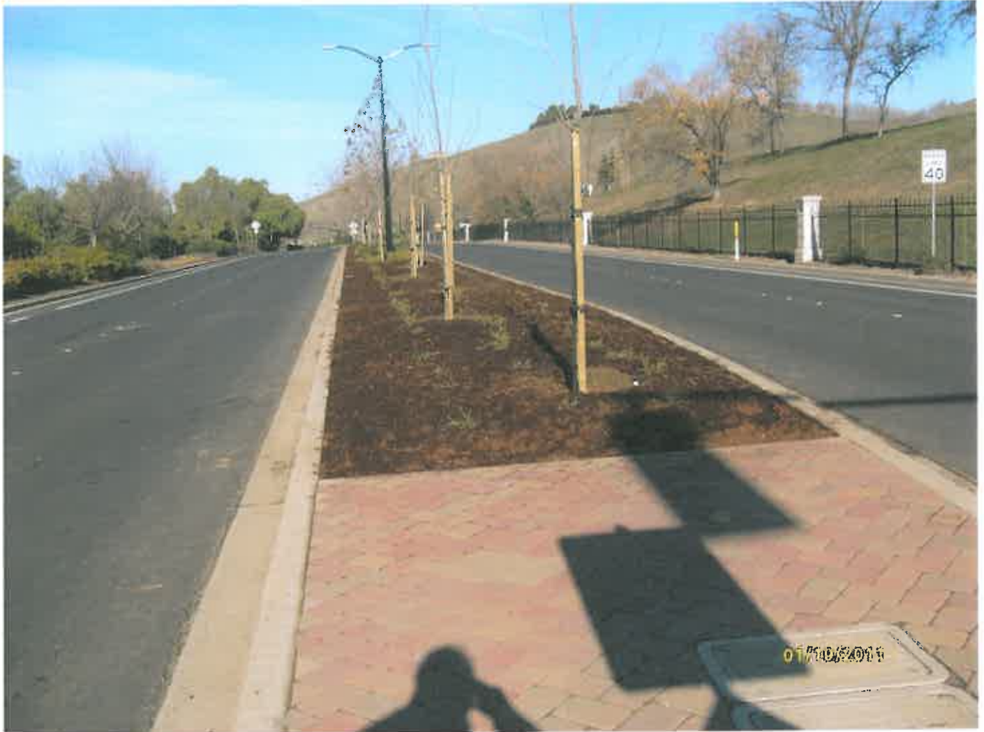
Oakhurst Blvd. -- Indianhead to Eagle Peak completed median: new hardscape/ new planting/infill planting and new irrigation
