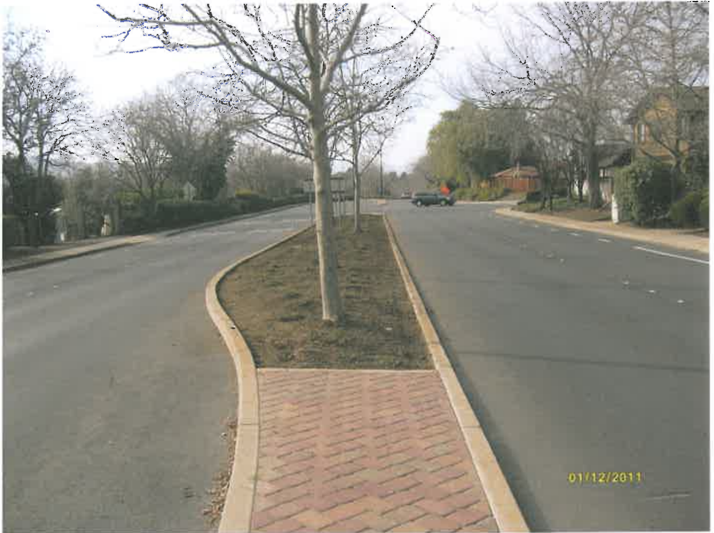
Oakhurst Blvd. -- Eagle Peak to Yolanda Circle completed median: new hardscape/new planting/relocated existing irrigation/new irrigation heads
